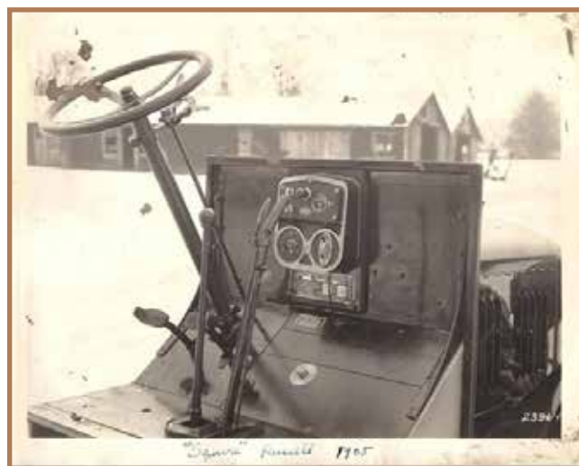
Two photographs from 1905 showing GMC truck detail. This photo shows the driver's controls
